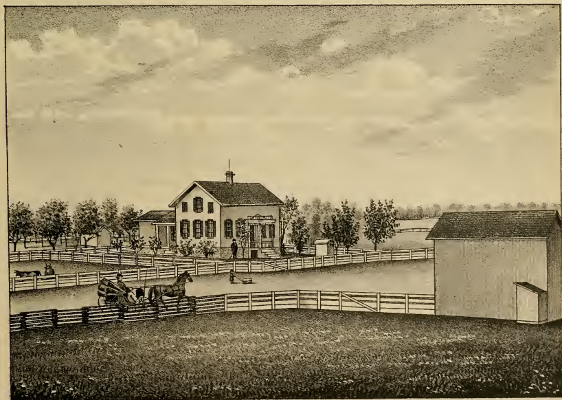
RESIDENCE OF JOHN BOWEN, NORWICH TWP., HURON CO., OHIO.
